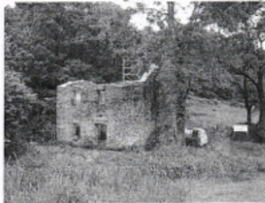
Noddon Mill during renovation 31 st July
